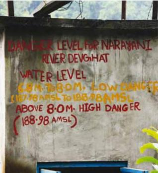
Left: typical image of Nepal, showing a river, terraces and erosion. In heavy rains landslides are common, in addition to river flooding. Right: shows flood levels on the side of a hydrological gauging station. These stations are permanently manned by an observer who takes care of the measurements and issues local alerts based on the river level and the instructions on the side of the building
