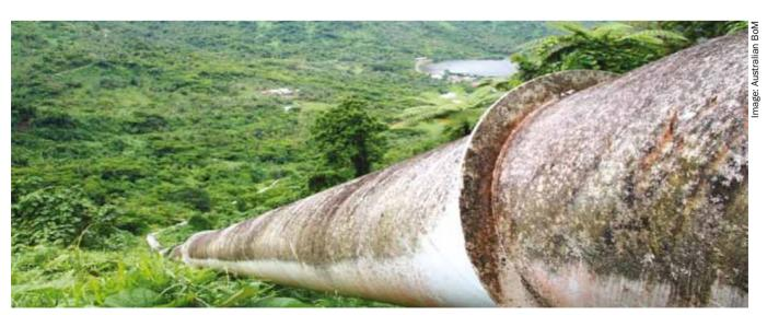
A penstock carries water from Afulilo Dam to the Ta'elefaga Powerhouse at Fagaloa Bay
