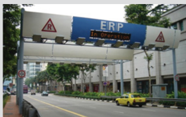
Figure B12.2.1 Electronic Road Pricing in Singapore
