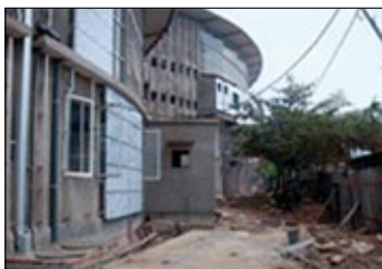
Figure 2: New bus terminal (target site) under construction in Negombo with Eco-Tank installation completed
