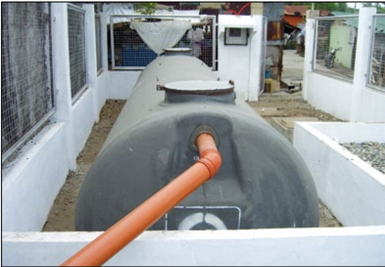
Figure 8: Eco-Tank installation completed in low-income riverside community
