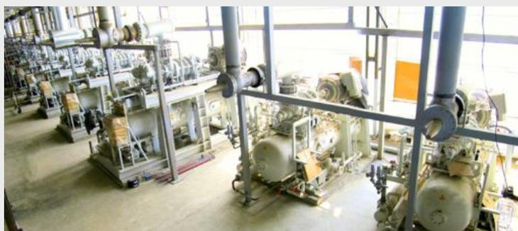
and processing purposes from -41°C up to -5°C. Excellent efficiency and performance results for single stage screw compressors reaching temperatures of -30°C or higher, and two-stage or compound screw compressors generating temperatures of -41°C, were obtained.
