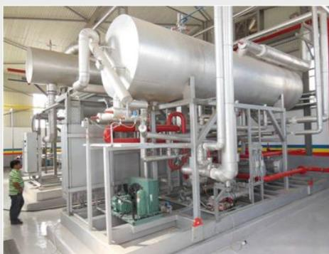
The products are frozen at a temperature of around -40°C in two air-cooled batch freezers. Also a chilling tunnel for cooling the freshly killed chicken uses CO<sub>2</sub> circulated at -10°C and a tunnel temperature about +1°C. A falling film ice water cooler is cooled with CO<sub>2</sub> at -10°C.
