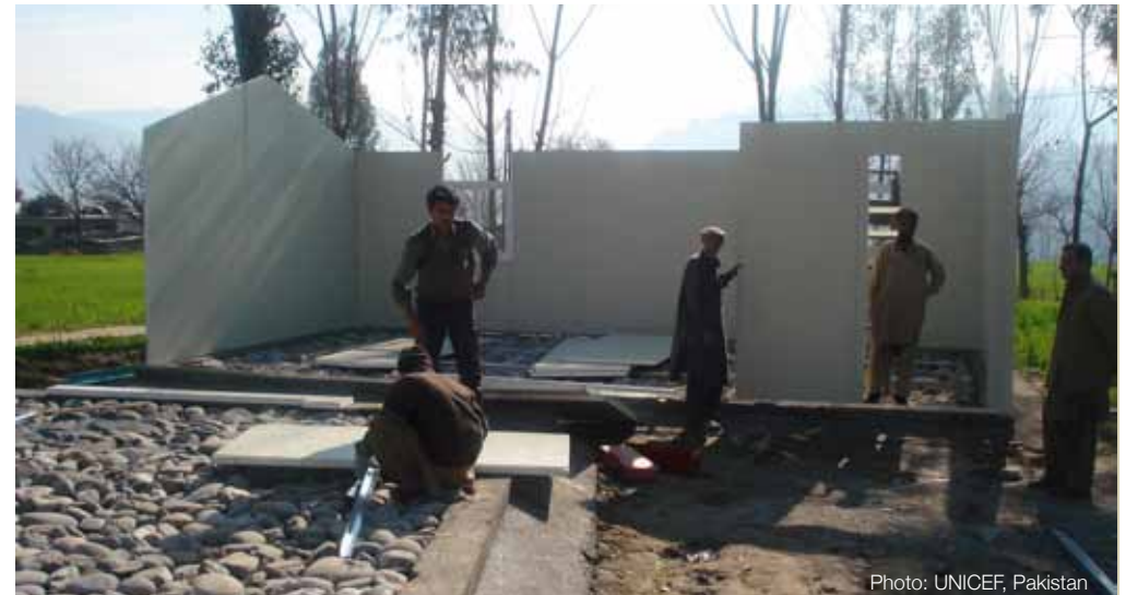
Assembly process of prefabricated wall elements
