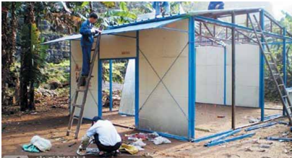
Assembly process of prefabricated classroom
