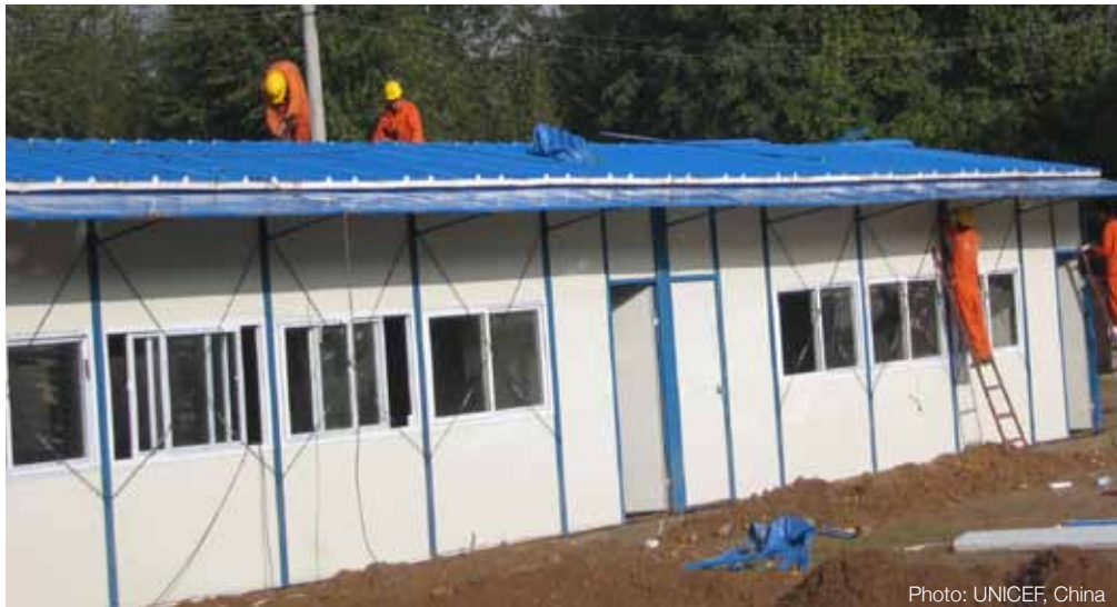
Assembly process of prefabricated school in Sichuan province
