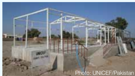
Photo: UNICEF/Pakistan Pakistan: raised floor level to prevent flooding
