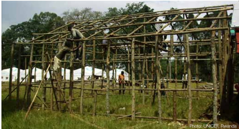
Wooden pole lattice structure, TLS under construction
