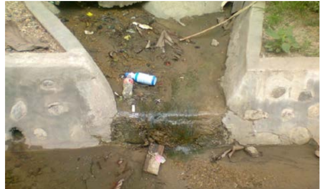
Drains blocked with soil and other waste materials in the Gordens Area Photo © Goiye, B., Kioma, T., Bobora, N., Bomai, A. and Kamaso, D. (2012)
