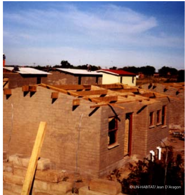
Stabilised Compressed Earth Block housing project, East London, Republic of South Africa
