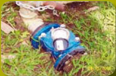
Tubigon, Philippines: Installation of flow meters at all water sources to achieve targets for potable water supply
