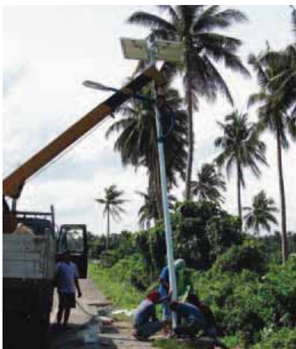
Installation of a solar-powered street light along Diversion Road in Sorsogon, Philippines © UN-Habitat/Joselito Derit
