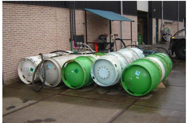
Photo 6-20 - One tonne (1000 kg) capacity pressurised cylinders
