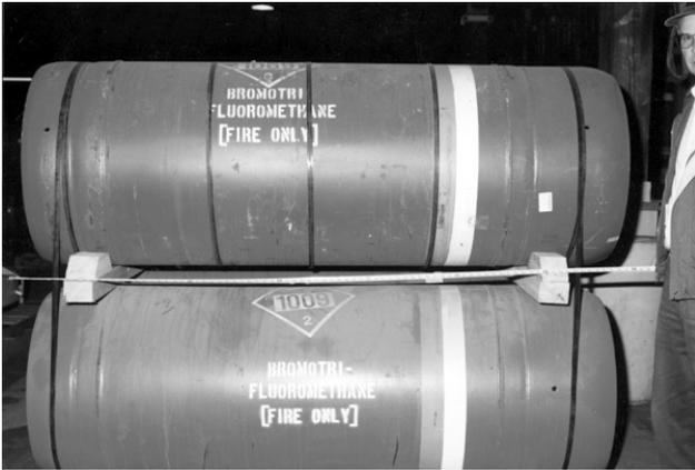
Photo 6-21 - Barrel of halon 1301 (bromotrifluoromethane).
