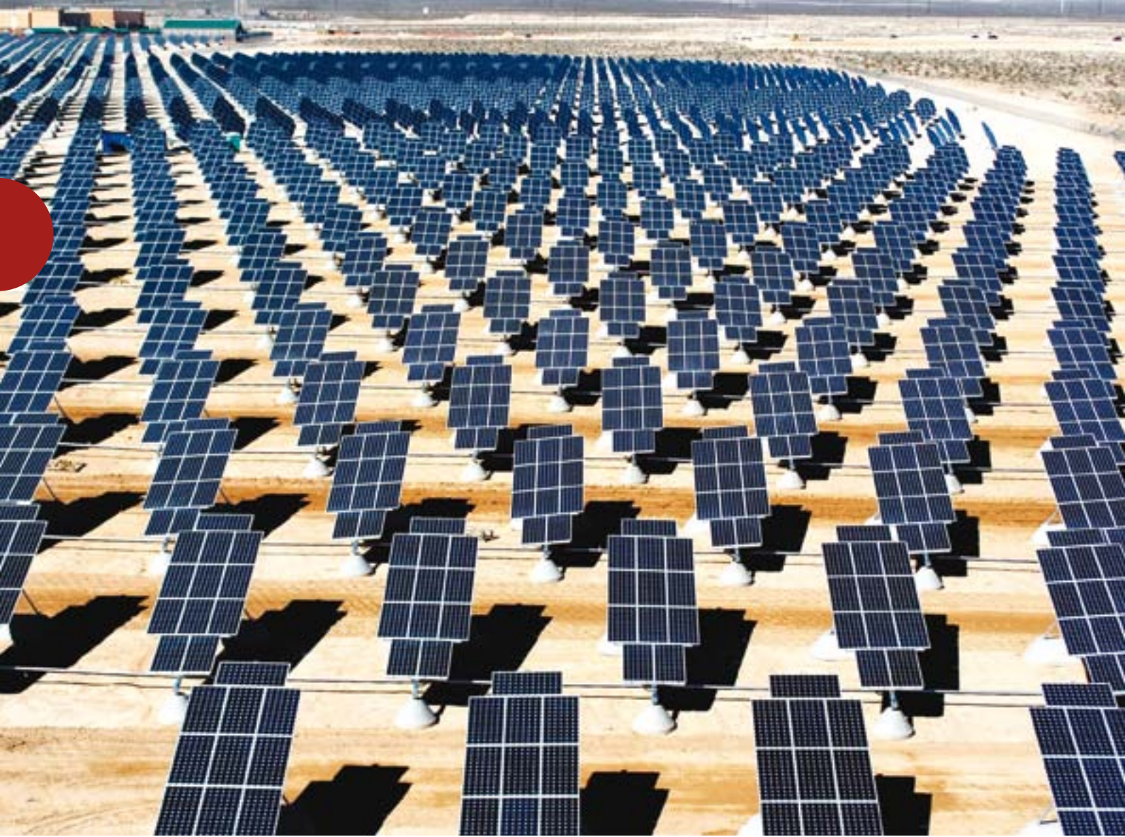
On 140 acres of unused land at Nellis Air Force Base, Nevada, United States, 70 000 solar panels are part of a solar photovoltaic array that will generate 15 megawatts of solar power for the base. Credit: Nadine Y. Barclay/USAF
