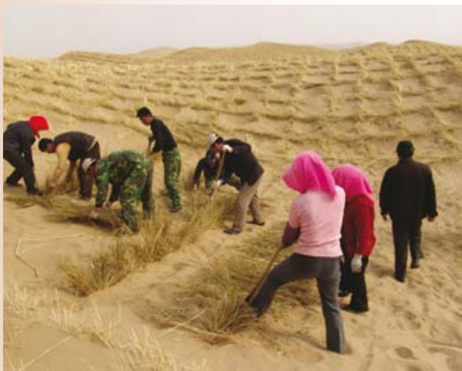
Sand barriers made of straw and rolled reeds are widely used to combat desertification in China. Semi-buried, and arranged in a checkerboard pattern, they stabilize the sand surface. Other techniques include planting grasses, shrubs and trees, excavating buried soils, and irrigation. Credit: Ningxia Forest Bureau
