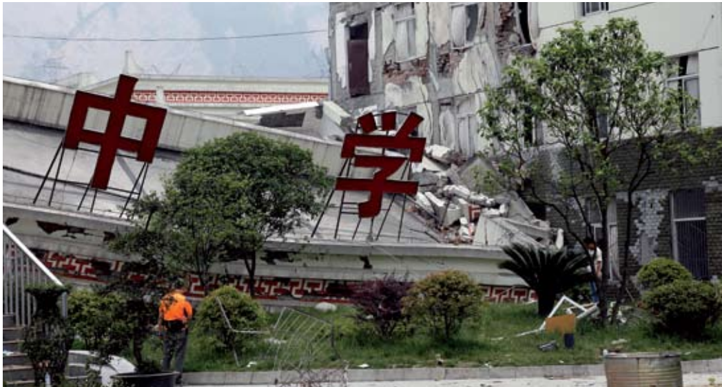
In Yingxiu Township, China, children were trapped when this Middle School collapsed during the 12 May Wenchuan earthquake. An estimated four thousand of the township's ten thousand residents died here at the earthquake's epicentre. Source: UN Photo/Evan Schneider
