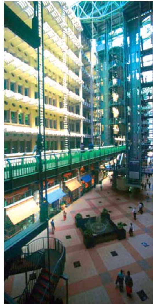
The Eastgate Building is designed to optimize climate comfort through the use of methods based on models from nature.
