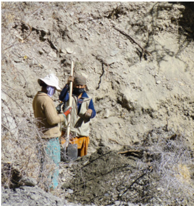
Digging an irrigation channel
