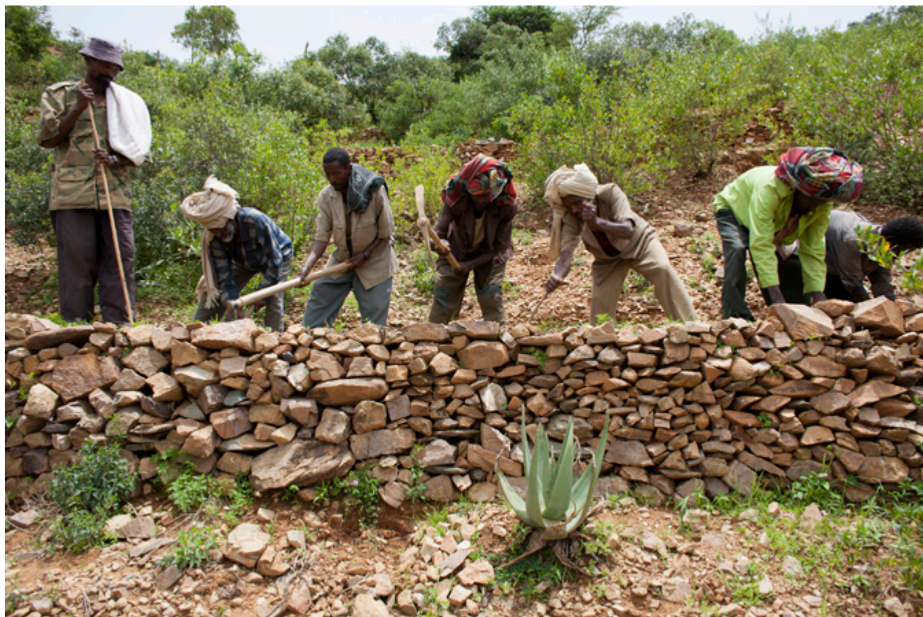
Rebuilding a dry stone wall to restore landscape functionality in Ethiopia
