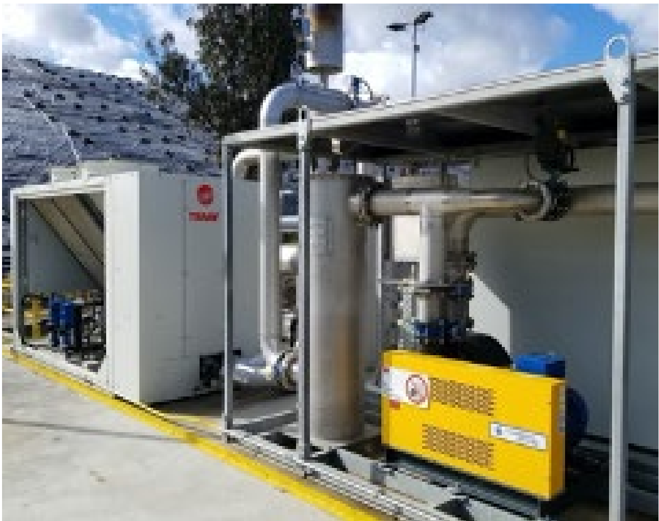
Figure 15. Copiulemu Landfill Gas Facility
