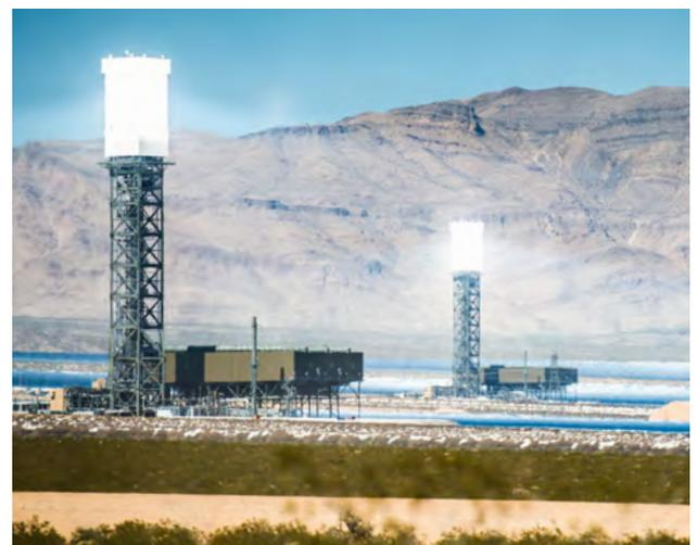
i Integrated Solar Combined Cycle facilities are hybrid gas and solar plants that utilise both solar energy and natural gas for the production of electricity.
