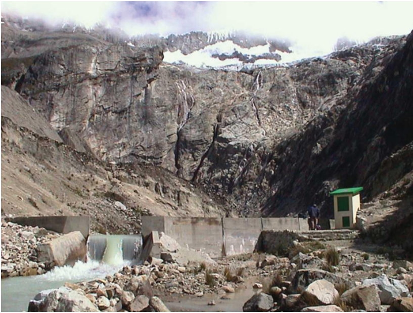
Figure A4.10. b) Hydrometric station installed at the outlet of Arteson Basin in the upper glacier
