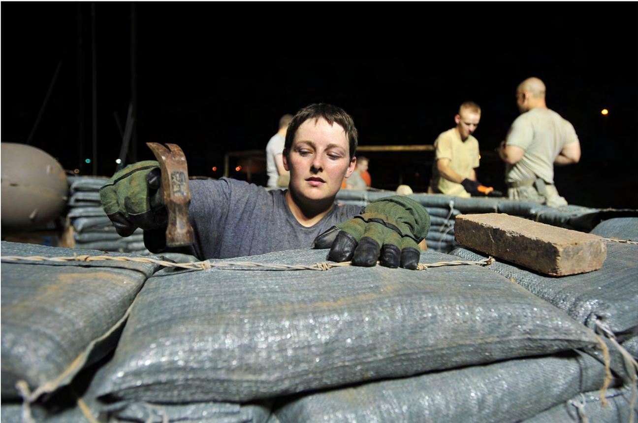
U.S. Army Sgt. Amanda Broome, Combined Joint Task Force-Horn of Africa Surgeon Cell animal care specialist, works on the construction of an Eco-Dome prototype. The Eco-Dome was engineered by the California Institute of Earth Art and Architecture to provide comfortable, economical and sustainable building solutions for impoverished and natural disaster stricken-areas. The design ensures the structure will be resistant to earthquakes, fire, flood and hurricanes.
