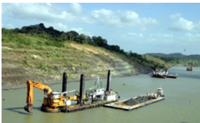
Figure 16: Dredging work in the Canal. Source: Emilio Mariscal
