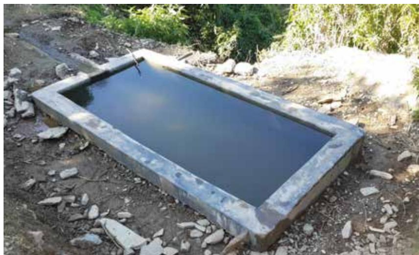
Rainwater is channeled into a catchment pit with concrete walls, allowing for infiltration and water use.
