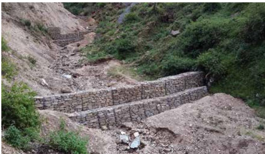
Community members built stone and gabion walls to prevent soil and water losses, and to reduce the impact of landslides.
