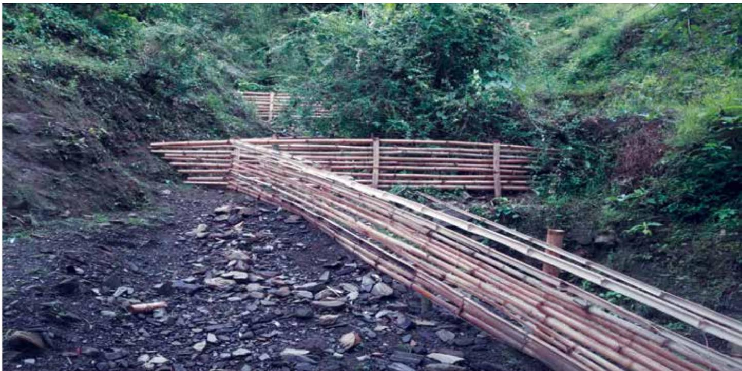
Using bamboo as vegetative check dams to prevent water run off and erosion loss down slopes, enhancing water infiltration and recharge.
