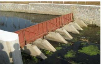
Figure 5. Water harvesting using flip-gates on drainage canal (left) and on-field (right).
