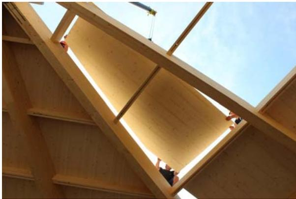
**Note:** Roof assembly with CLT boards on a glued laminated timber primary structure.
