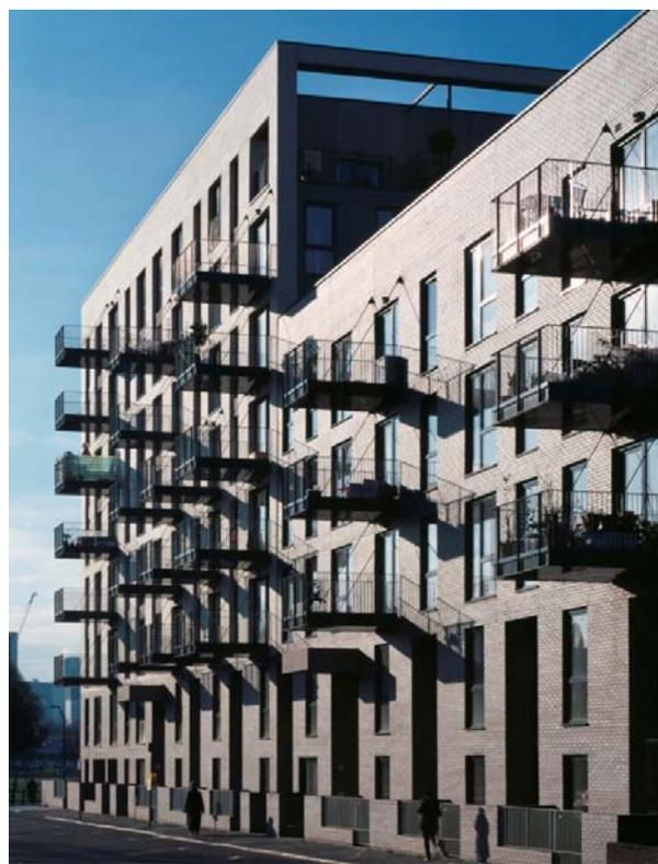
**Note:** 1,198 tonnes of stored CO<sub>2</sub> equivalent: the largest solid timber building in the UK, "Bridport House".
