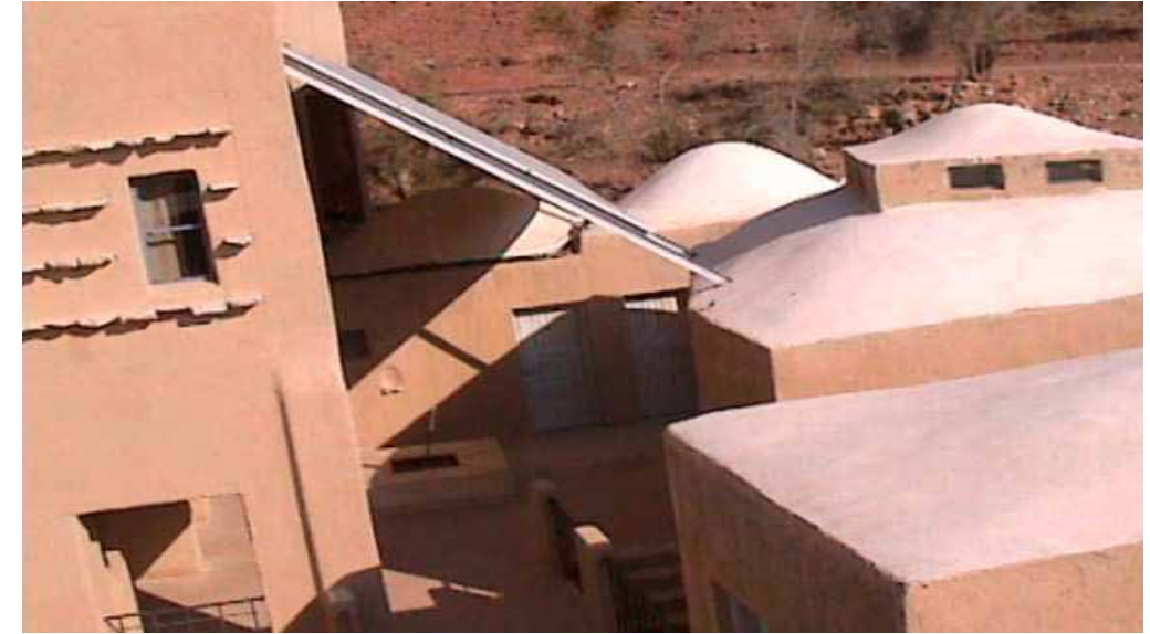
Figure 6. PV modules for shading
