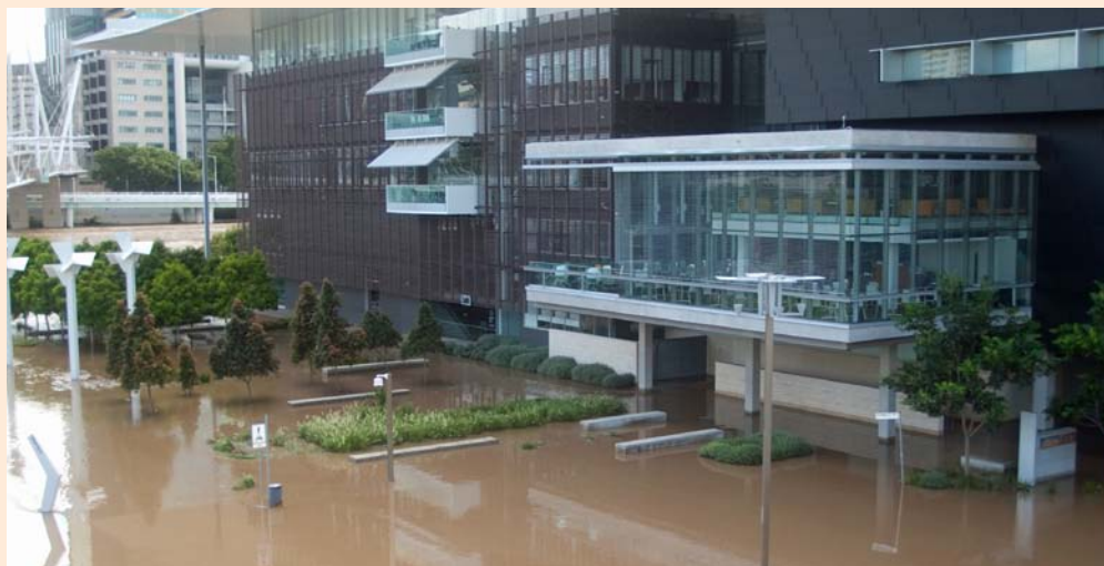
Central Brisbane, Australia, during the 2010-11 Queensland Flood. This event prompted changes to land-use planning and building codes in the State © Wikimedia Commons/ Rae Allen
