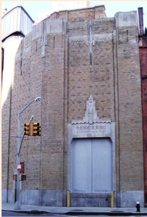
The 13 th West Street electricity substation in Manhattan, USA, which was flooded during Hurricane Sandy in 2012.
