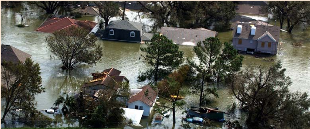
An aerial view of flooding in New Orleans, USA, a day after the levees failed. On 29 August 2005, storm surge from Hurricane Katrina caused 53 different levee breaches in greater New Orleans.
