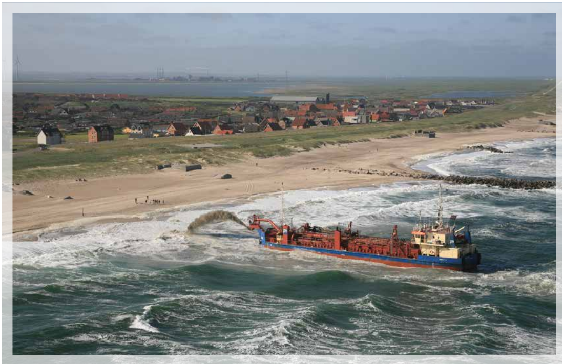
Fig. 1.2. Beach nourishment with Trailing Suction Hopper Dredger and Rainbowning method for transferring nourishment material ashore. Slurry is discharged via a jet at the bow of the ship once it has been sailed as close to the shore as possible (Photo: Rohde Nielsen).
