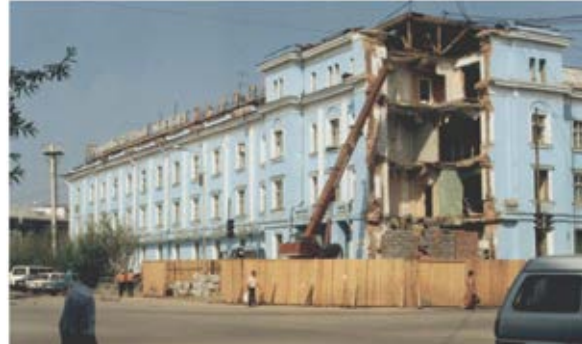
Fig. 2.8.11. The collapsed corner of a building in Yakutsk (Russia).
