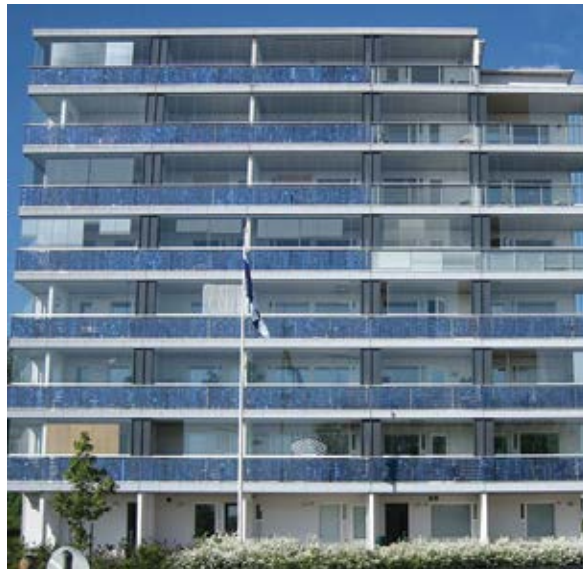
Fig.3.2.11. A number of low-energy buildings have been constructed in the Viikki district of Helsinki (Finland). Panels that store energy from the sun have been built into the facades.
