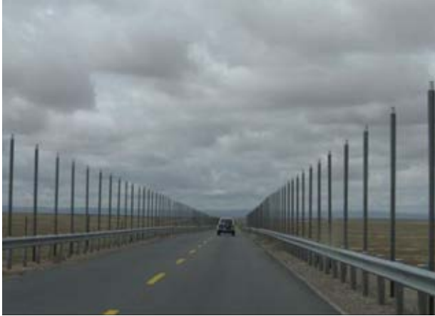
Fig. 2.8.13. Road with soil-freezing thermosiphons.
